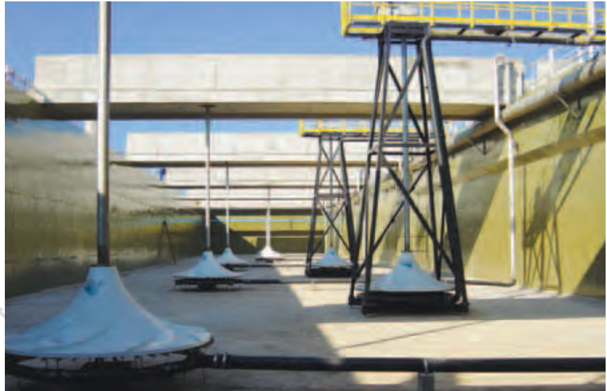
8 out of 22 HYPERCLASSIC® -Mixer/Aerators in a large municipal wwtp in Sao Paulo, Brazil
