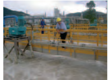
5 HYPER-CLASSIC® Mixing & Aeration Systems in an industrial wwtP in Brazil (Chemical Industry)
