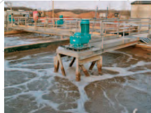
4 HYPER-CLASSIC ® Mixing & Aeration Systems in an industrial wWtp in Belgium (Food Industry)
