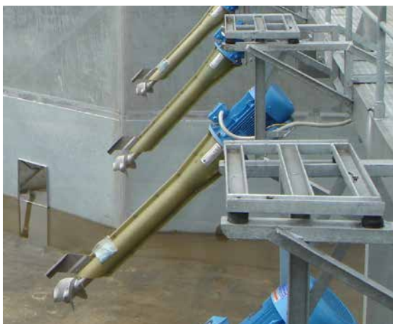
OxyStar® aerator on standard mounting bracket
