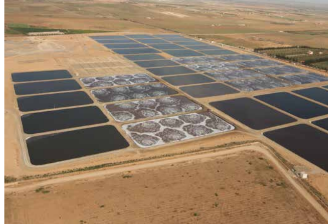
Aerated wastewater lagoon system with OxyStar® aerators (Morocco)
