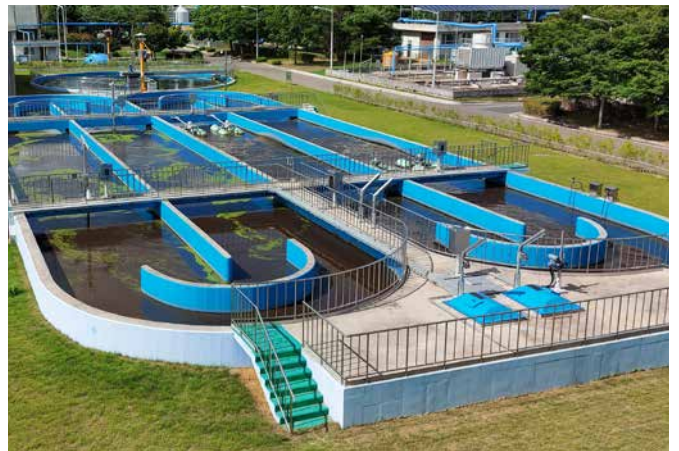
Oxidation ditch of a municipal WWTP (Korea)
