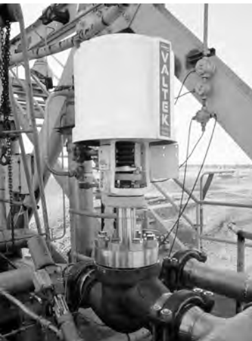
This cryogenic Mark One is used for aerospace testing as an O 2 vent.
