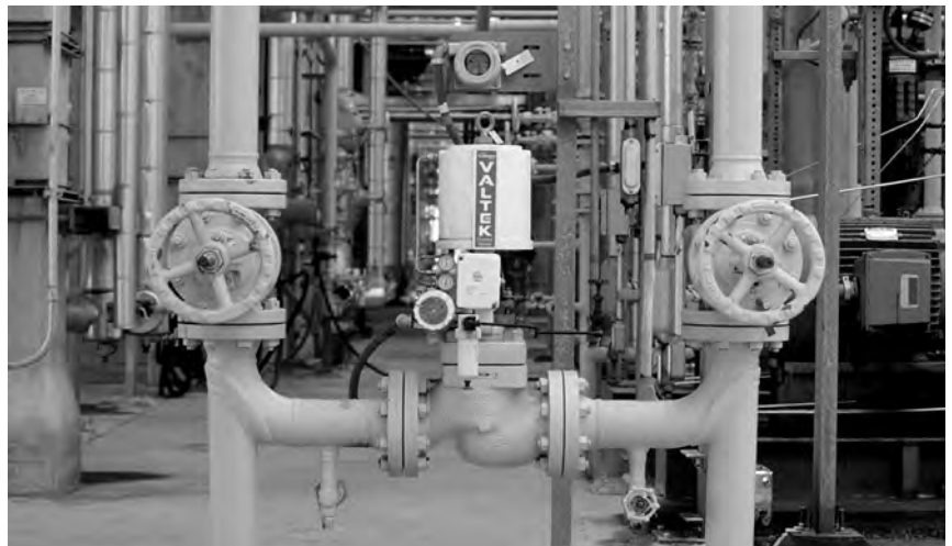
This 8-in, back-pressure control valve operates in a liquid hydrocarbon plant with a 580 psi/40 bar upstream pressure.
